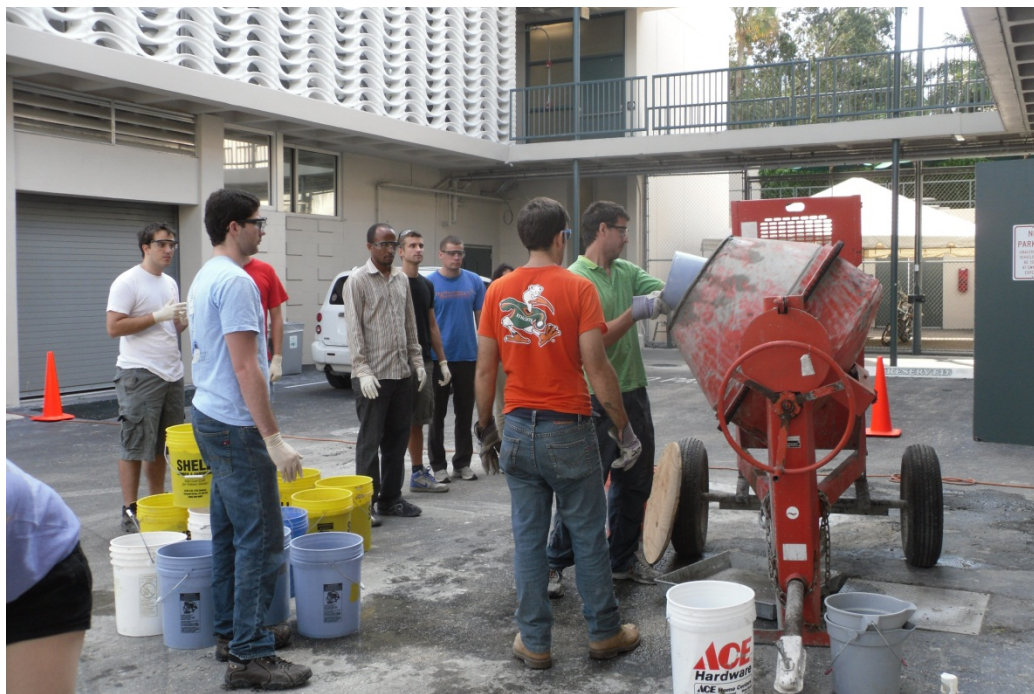
Figure B-3 - Concrete mixing with 9 cubic foot mixer
